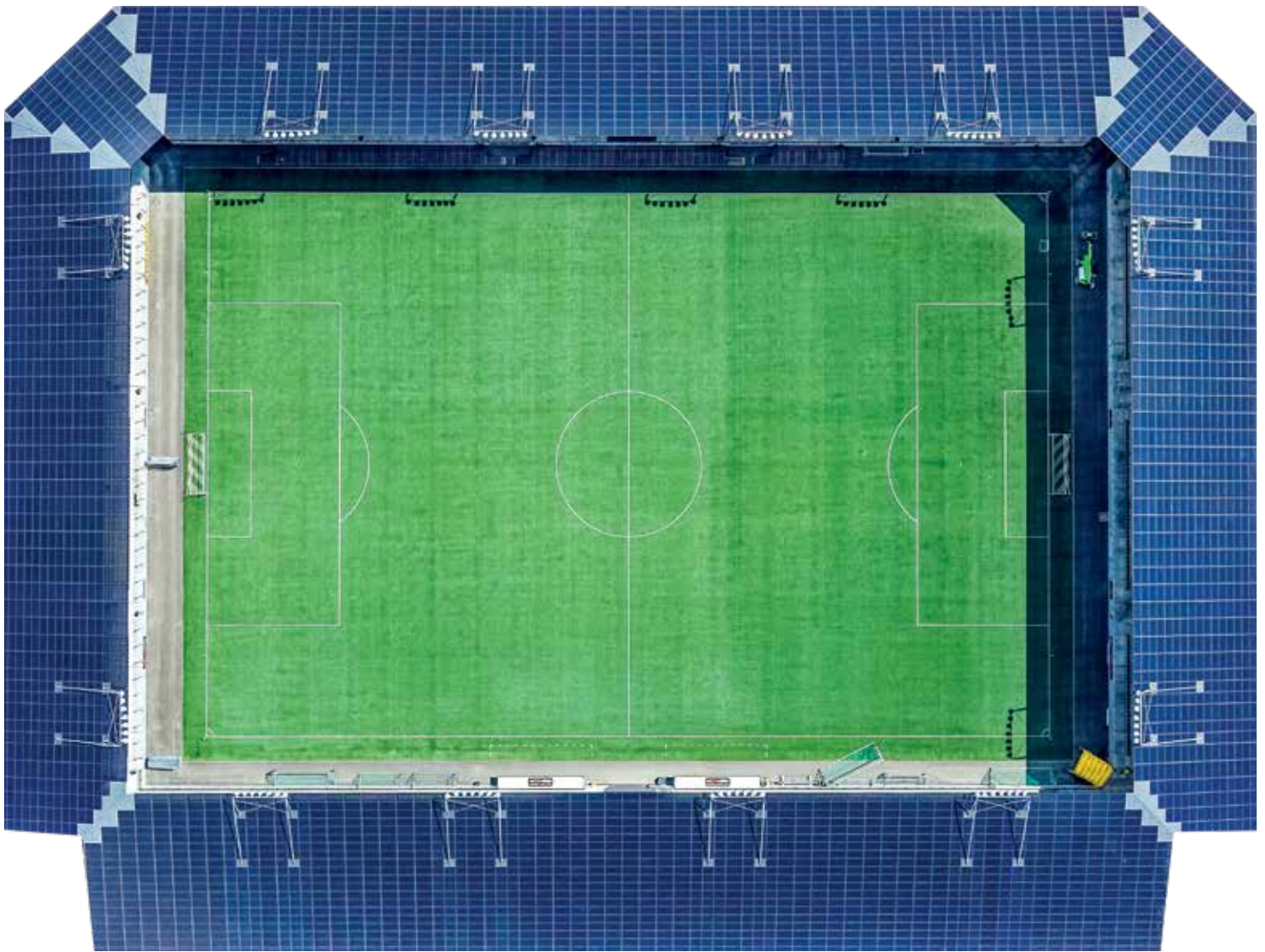
150%-PlusEnergie-Fussballstadion Lipo Park, Schaffhausen
