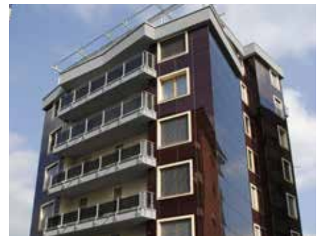
NFSA-Diploma: Palazzo Positivo, refurbishment, Chiasso/TI
