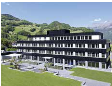
Flumroc office building refurbishment, 8890 Flums/SG
